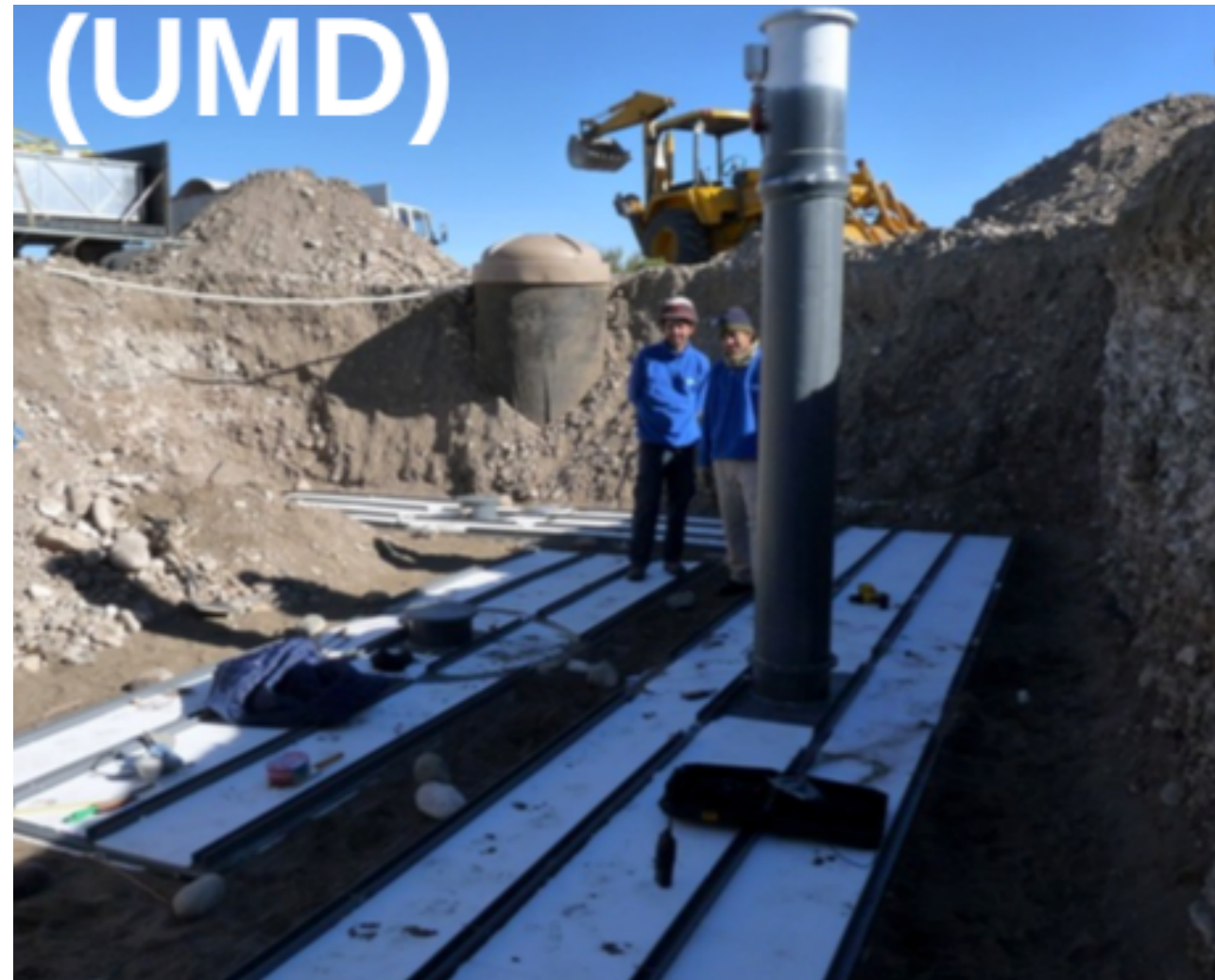
Underground muon detectors (2.3 m soil for shielding)
