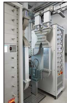
RF amplifier for FZD 10kW @1.3 GHz
